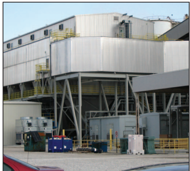
Figure 7: Typical baghouse from an electric power plant
