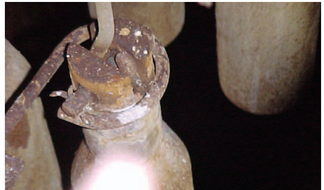
Figure 7: Alignment ring should be below the rivet pin to account for wire lengthening when on-line.
