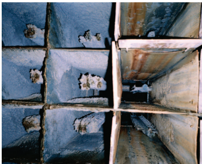
Figure 8: Membrane build-up test at NSP's Sherco Station
