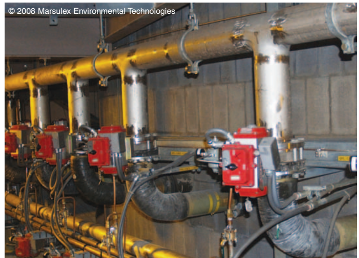
Figure 19: Mist Eliminator Wash Headers.
