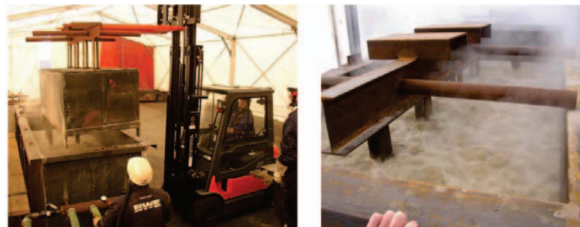
Figure 19: Washing of catalyst modules at Studstrup Power Station
