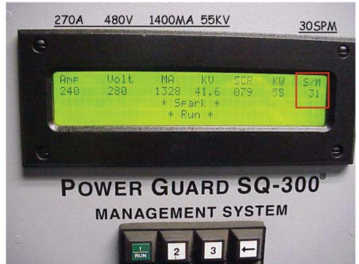
Figure 17: AVC spark Limited – doing its job. The actual T-R set rating is shown on top and the actual ESP operating values are in the green.
