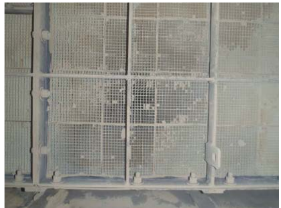
Figure 36: After Ice Blasting
