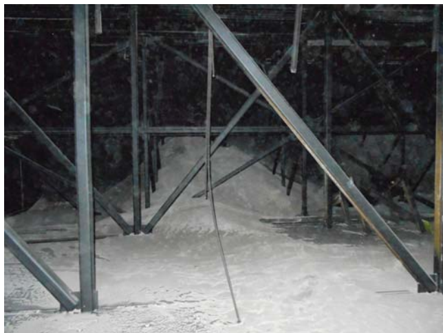
Figure 1: Typical accumulation of flyash in a coal-fired power plant duct
