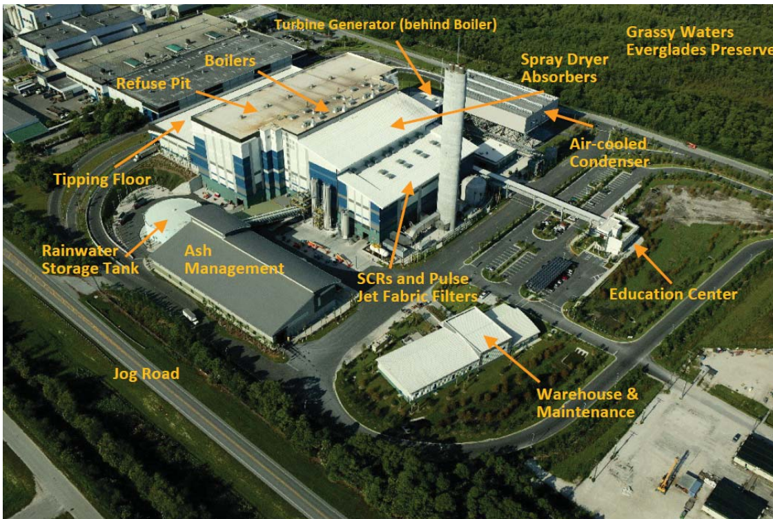
FIGURE 23: PBREF No. 2 plant overview (from June 2015 looking from northeast to southwest).
