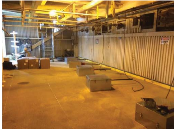
Fig 25: Sorb-Tec Injectors on B Duct prior to installation (sound enclosures shown).
