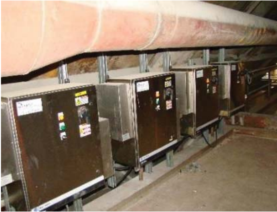
Fig 19: Image of Variable Frequency Drives (VFD) installed on a major utility-scale coal-fired power plant
