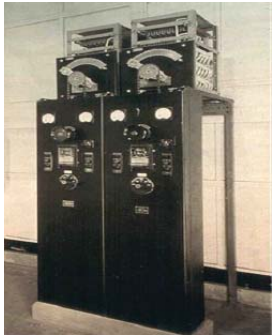
Figure 32: Variac and rheostat control
