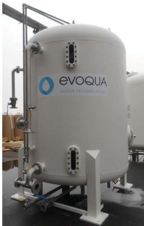
Figure 28: WWIX Exchangeable Resin Bed
