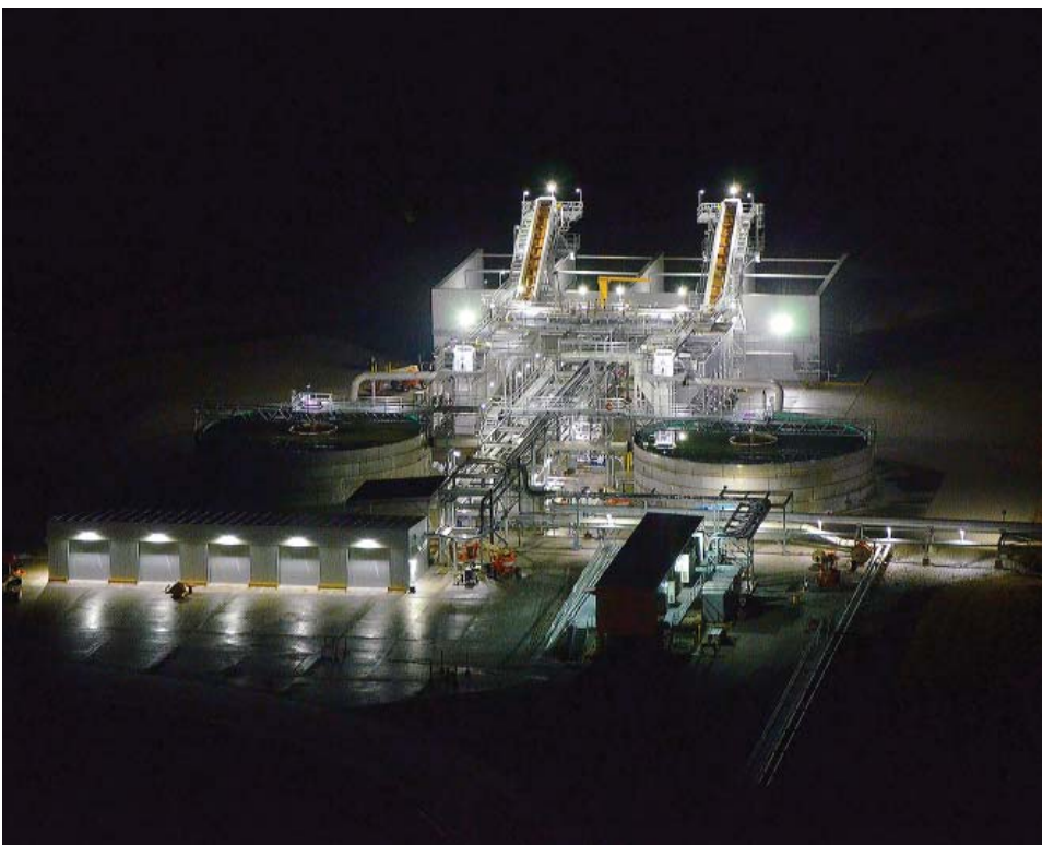
Figure 3: CDR System at night.
