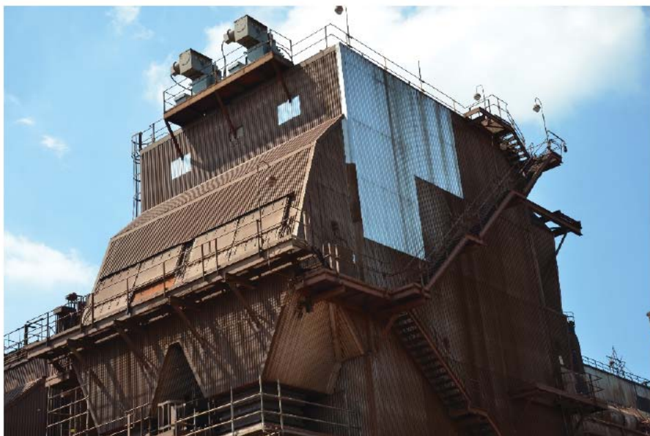
Figure 27: Modifications and additional space required for ESPs
