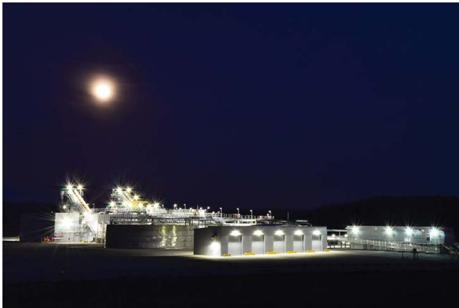
Figure 1: CDR System at night.
