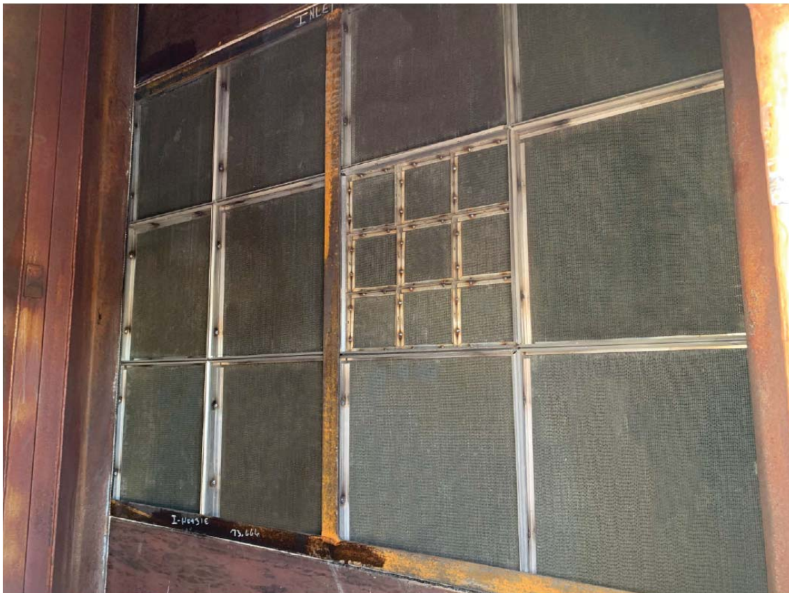
Figure 3: Umicore's TripleCat catalyst with test elements installed in a US based boiler, the darker color of the catalyst compared to standard DNX catalyst is due to the much higher vanadium loading.
