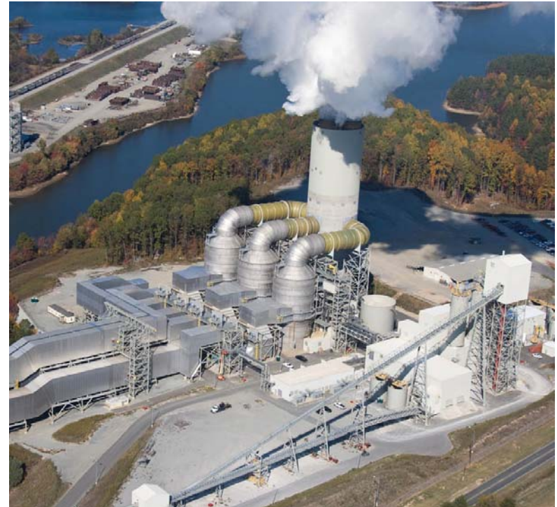
Duke Energy Marshall Units 1-4 Terrell, NC
