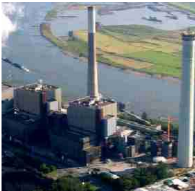
STEAG's Voerde Power Station
