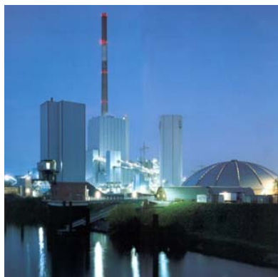
STEAG's Walsum Cogeneration Plant
