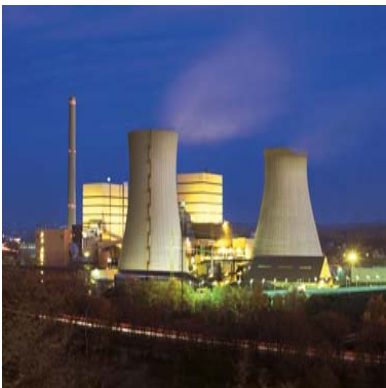
STEAG's Fenne Cogeneration Plant
