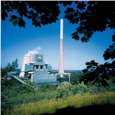
STEAG's Bergkamen Power Station
