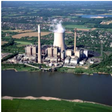
STEAG's Voerde Power Station
