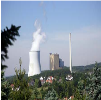
STEAG's Bexbach Power Station
