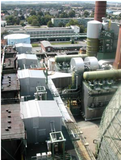
STEAG's Godorf Cogeneration Plant
