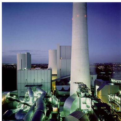
STEAG's Herne Cogeneration Plant
