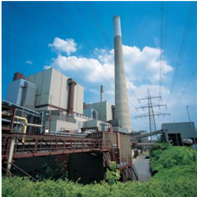
STEAG's Voerde Power Station
