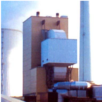
STEAG's Bexbach Power Station
