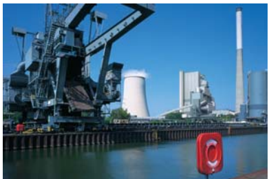
STEAG's Bergkamen Power Station
