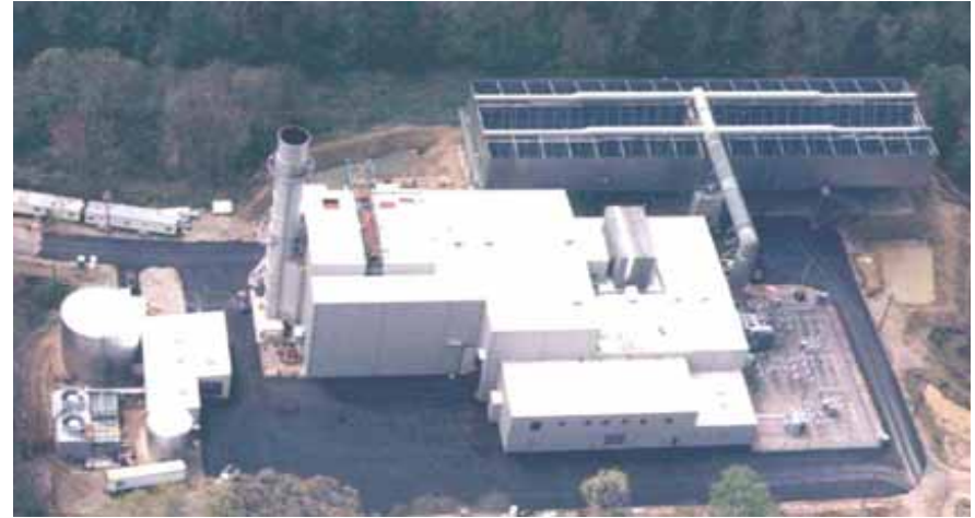
Gas Turbine – Over 33,000 MW
